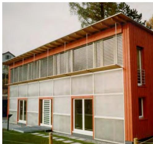
Fig. 3-1: Basic types of TI systems: Direct gain or light wall (top), and solar wall (bottom). Bottom left:
